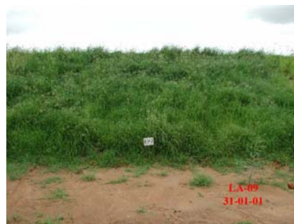
Fig. 10. Laleham site. Drip lines were laid on all batter sections at row spacing between 1 m and 2 m
