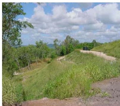
Fig. 12. Black Mountain Derailment Site. Drip lines were laid on all batter sections at row spacing from 1m to 2 m.
