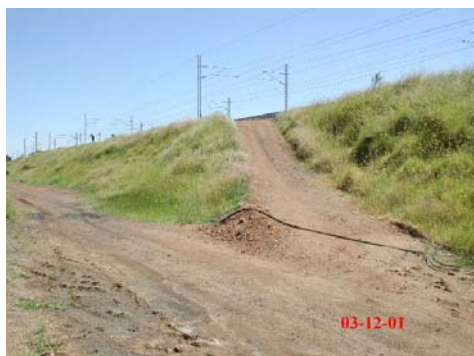
Fig. 11 Riverside Mine site. Drip lines were laid on all batter sections at row spacing between 1 m and 2 m.
