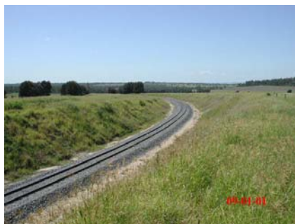
Fig. 9 Boundary Hill Site. Drip lines were laid on all batter sections at row spacing between 1 m and 2 m
