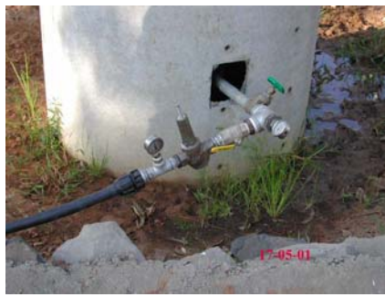
tapping existing pressurised water mains (at scour valve)
