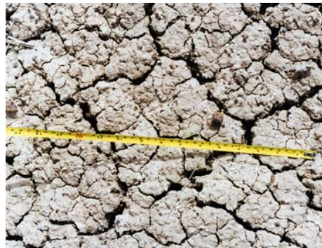
cracks on surface sealed batter
