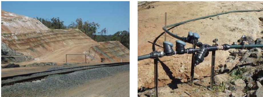
Fig. 6. Holmes cutting site – lowest two batters showing emitter wetting fronts (left) and the irrigation control valves (right).
