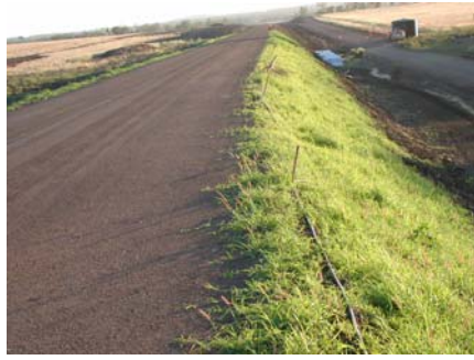
Fig. 13. Bauhinia Site. Grasses established before track was laid. Three rows (1 m spacing) of drip lines were laid at the top batter section only.
