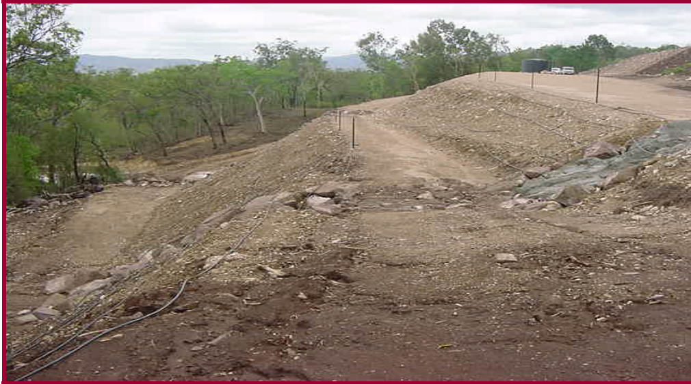
Freshly constructed batters (Black Mountain)
